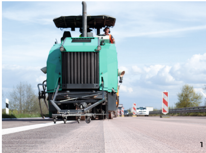
1 Production lane to lane - patented control technology via scanning | 2 Grinding/grooving shaft - variable composition for optimised surface design | 3 modern measuring and control technology - increase in process/product quality
