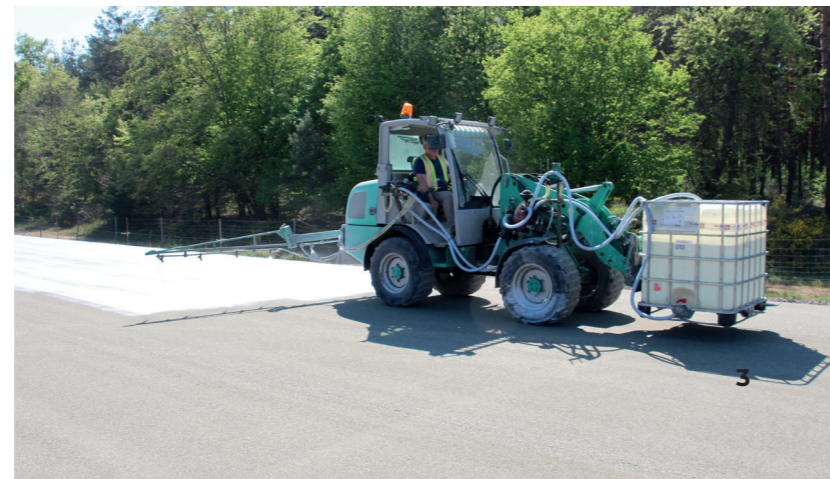
1 variable working width up to 10 m | 2 specific spraying system depending on applied material | 3 applying on all kind of concrete pavements
