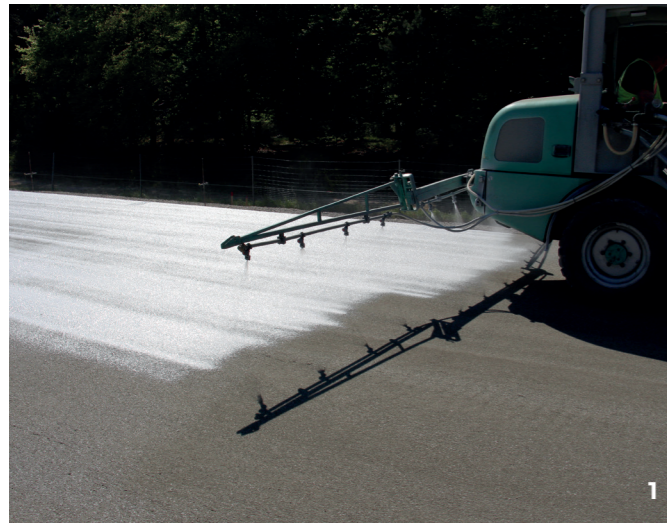
1 variable working width up to 10 m | 2 specific spraying system depending on applied material | 3 applying on all kind of concrete pavements
