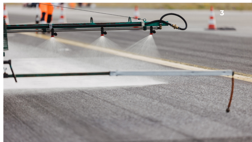
1 Onyx application | 2 digital adjustment of the application quantity | 3 eshabit Onyx Primer as a bonding agent
